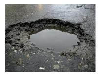
For a carriageway a pothole has been defined as a sharp edged depression anywhere in the carriageway where part or all of the surface layers have been removed including carriageway collapses, surrounds to ironwork and missing cat's eyes. A pothole will be identified when its maximum horizontal dimension is greater than 250mm and is:
